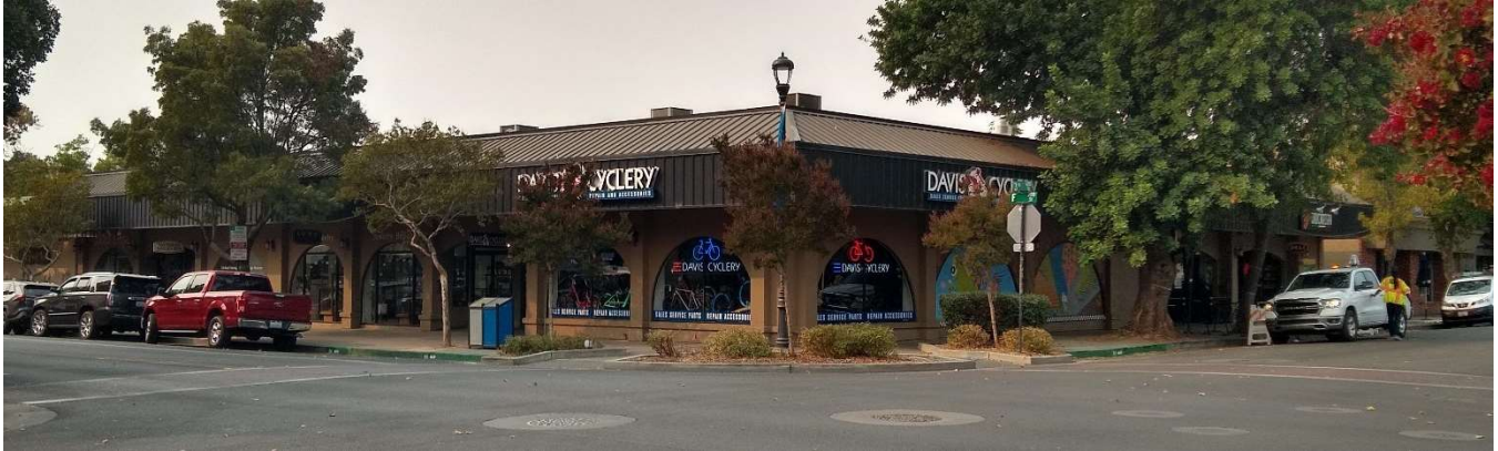
East and north facades, looking southwest, ESA 2022.
